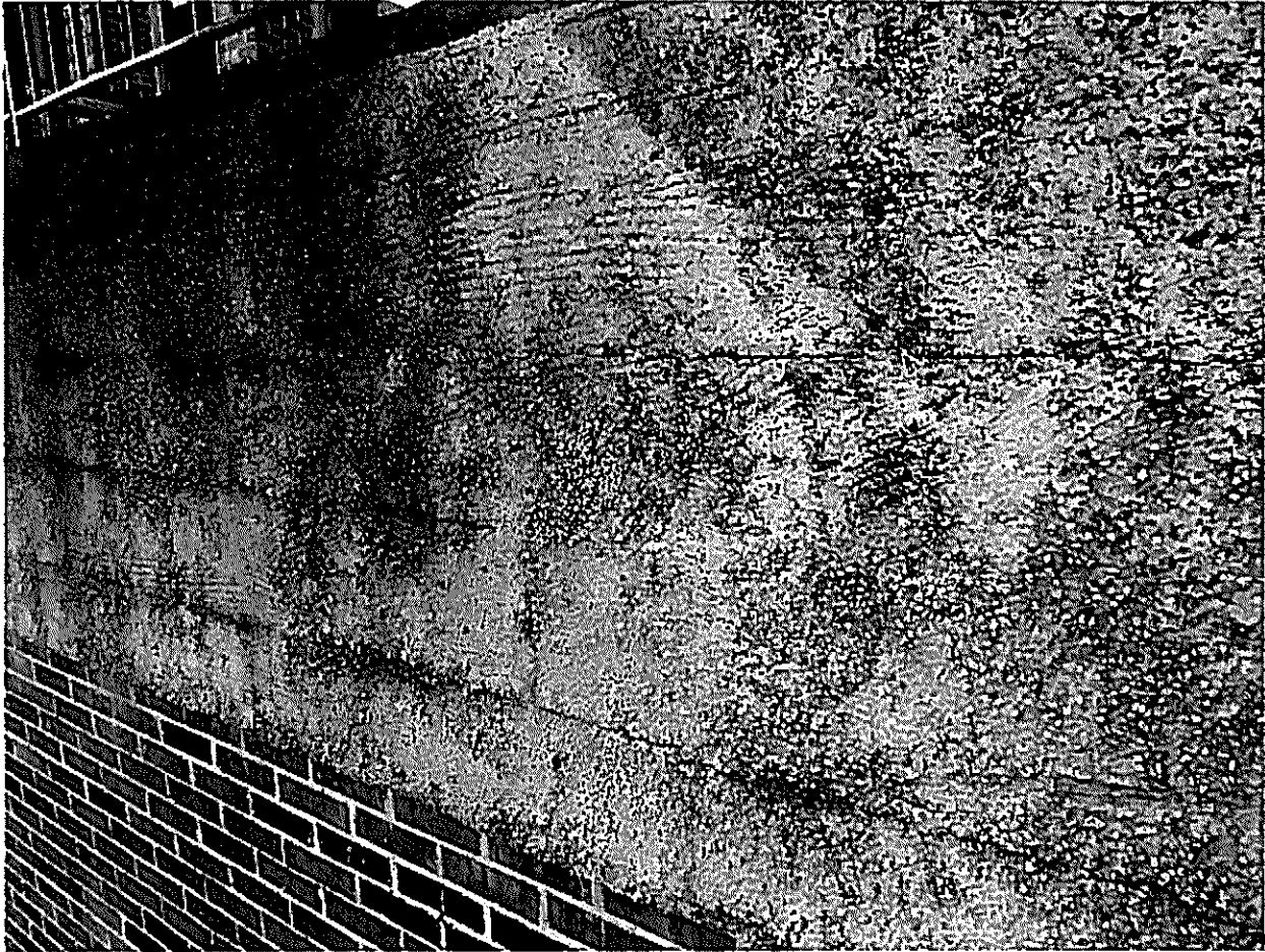
Discoloration and cracking on coping.
