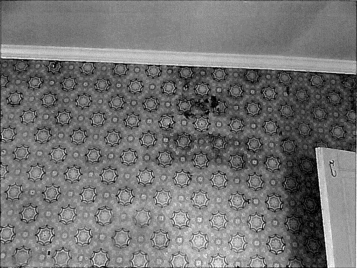
Possible mold starting due to moisture issues.
